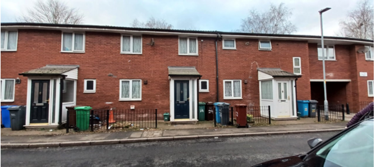
Figure 3. Photograph of the principal elevation of No.24 Victory Street.
