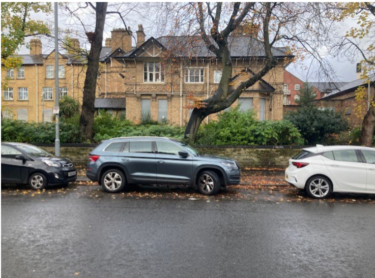
View of existing buildings from Oxford Place
