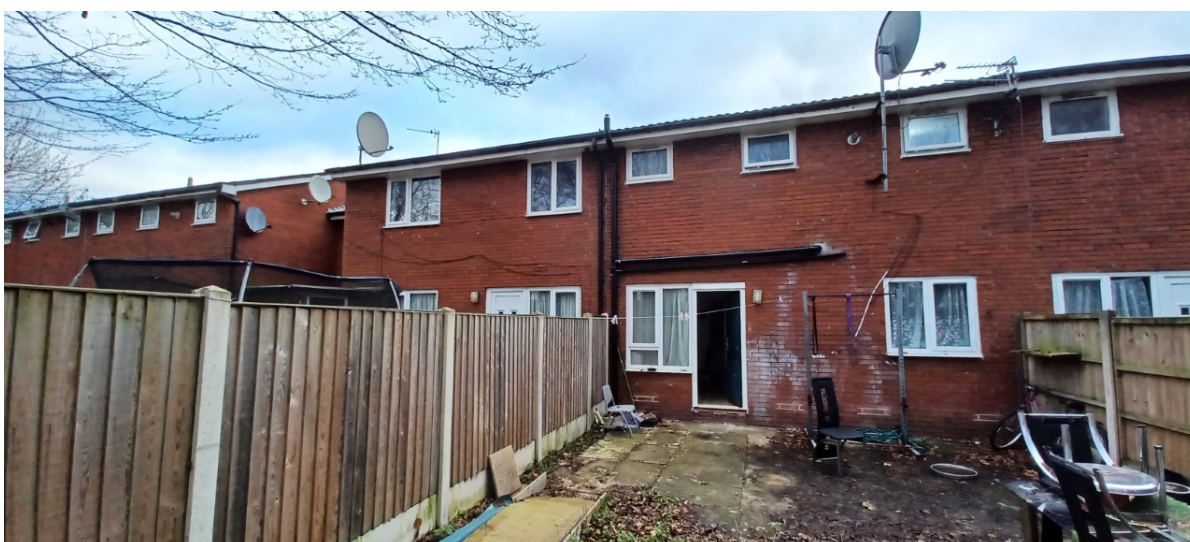
Figure 13. Photograph of the rear elevations of No.24 and No.22 Victory Street.
