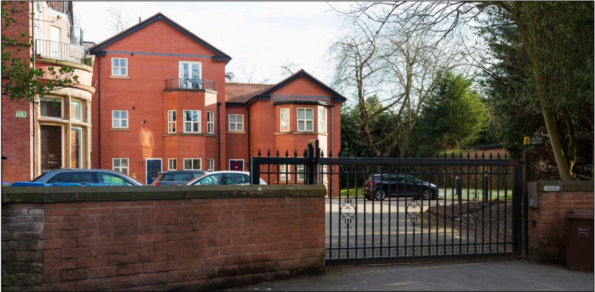
View from Holme Road of existing Cairncroft building which neighbours the site to the west
