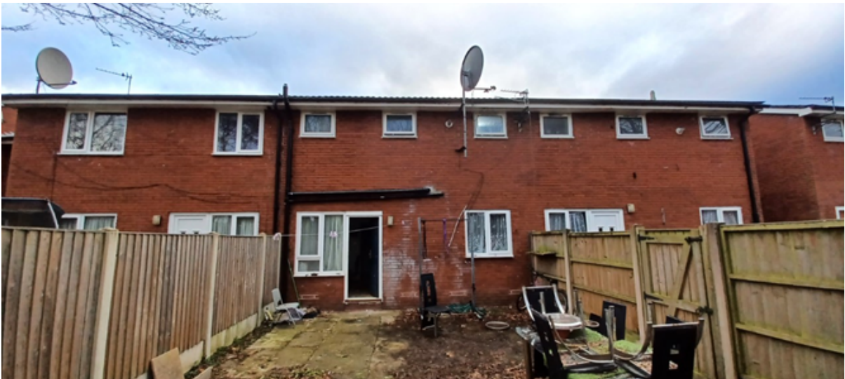
Figure 4. Photograph of the rear elevation of No.24 Victory Street.
