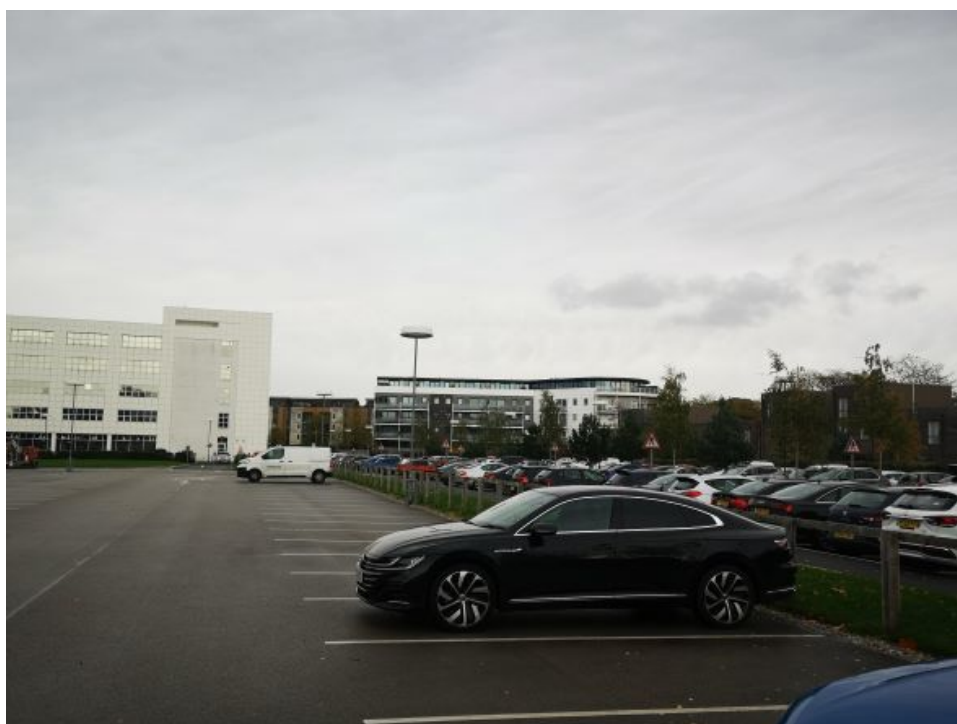
View North across existing surface car parking towards the recently developed apartment block to the right and Sir William Siemens House to the left
