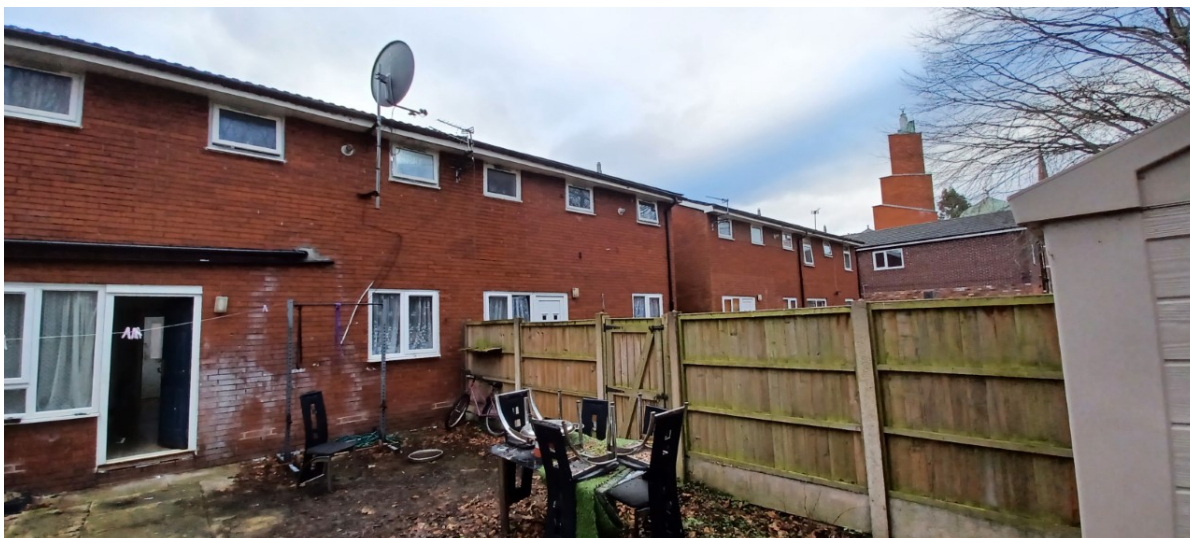
Figure 12. Photograph of the rear elevations of No.24 and No.26 Victory Street.
